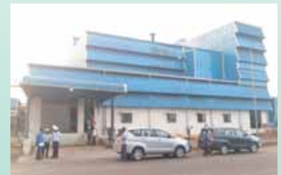
SSP "POME to Animal feed" plant at Godrej Palm Oil Mill
